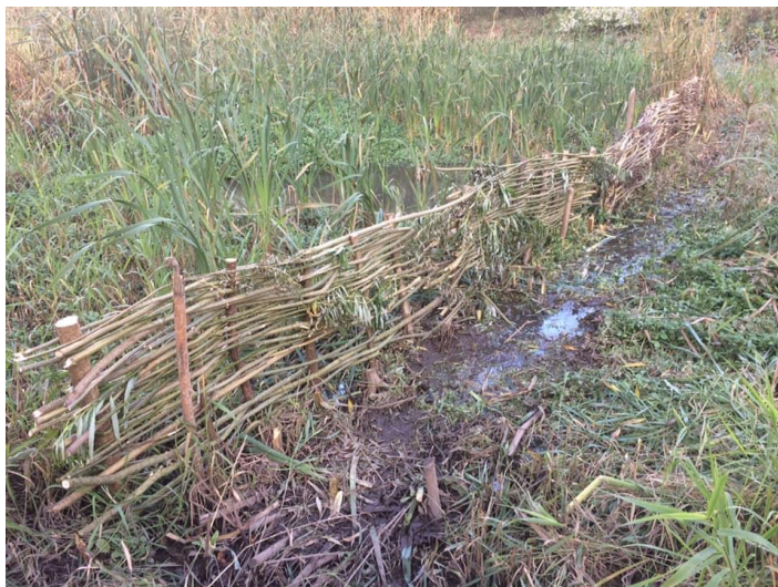
Progress with hurdles forming the dam.
