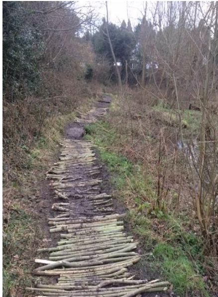
Improvements to the path using fallen Ash limbs.
