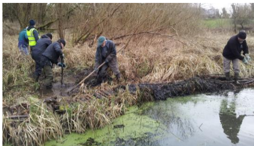
Digging a new pond.
