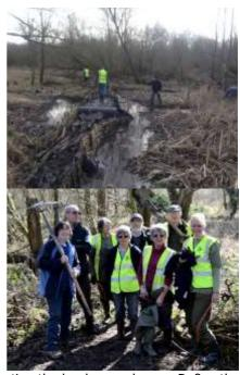
Working Party Activity (2). Reed bed creation the hard manual way. Define the area, build retaining hurdles, insert a pipe, build up an access route. Then shovel the silt and other unwanted material – Good clean fun! (Photos: AN, PRE, PC).
